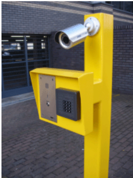
Bullet IR camera on a barrier pedestal
