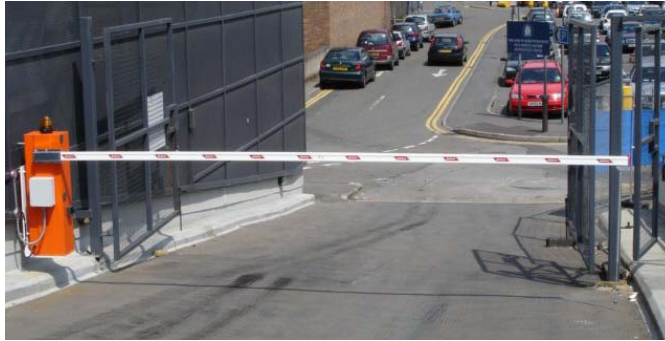
Automatic Traffic Barriers
